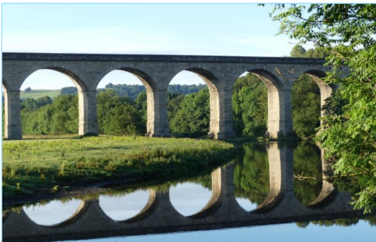
Arthington Viaduct, West Yorkshire Photo: Steve Davey @Wharfephotos
