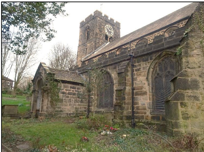
South Windows with conifers removed
